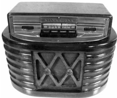
Silvertone model 6320 radio – Manufactured in 1938 by Sears. Cabinet is wood with metal escutcheon. There are four pushbuttons. Chassis is mounted from bottom. Chassis number 101.585. Steven Kirschner, Atlanta, GA
